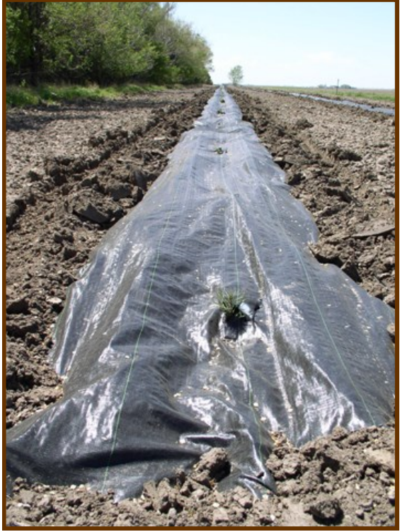
Tree Planting and Weed Barrier Installation
